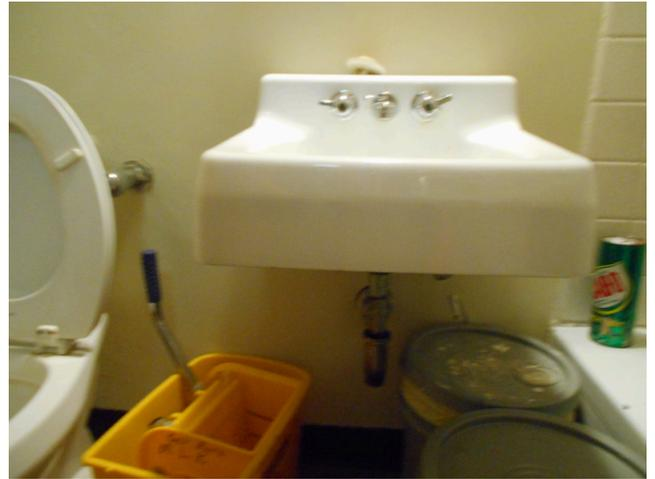
6. 0br/1ba, Unit 7 - Bathroom sink, no scald abrasion protection
