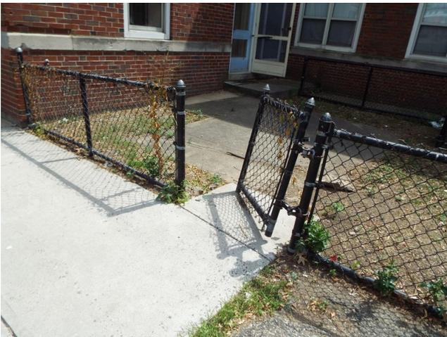
423. Building 10 - chain link fence damage (Non-Critical Repair)
