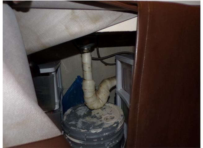
198. Building 7 - unit 735 - 2-bed/1-bath - UFAS - kitchen sink missing scald and abrasion protection (Critical Repair)
