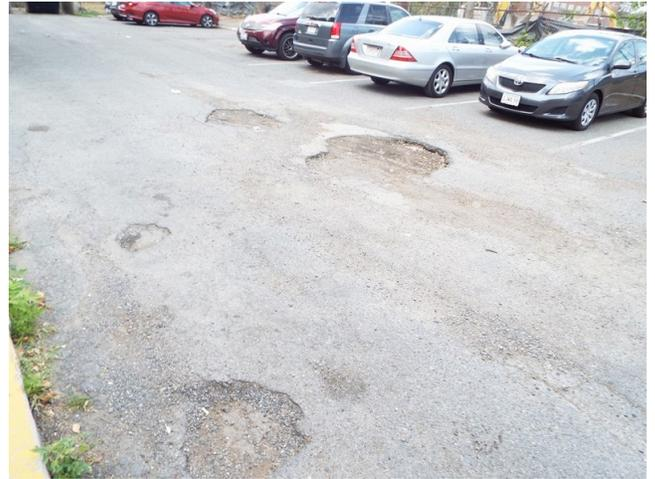
430. Building 10 - asphalt parking lot condition (Non-Critical Repair)
