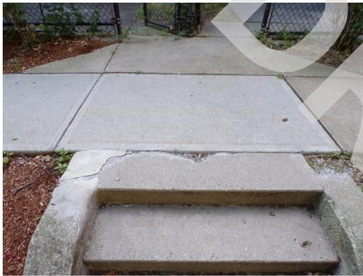
Building 4 - concrete trip hazard (Critical Repair)
