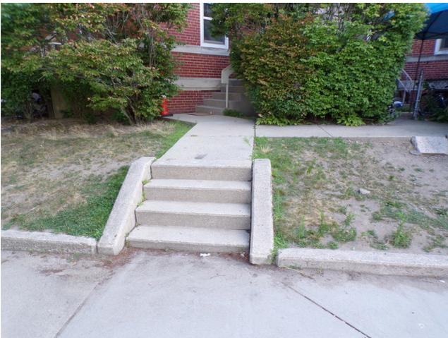
39. Building 4 - concrete stairs missing railing (Critical Repair)
