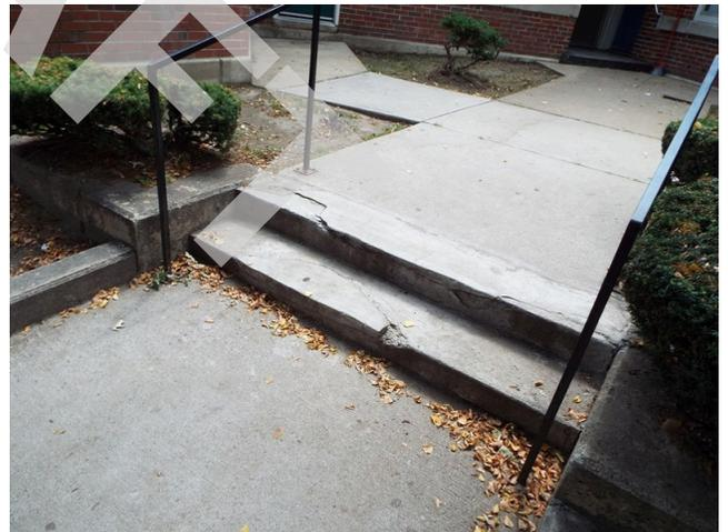
448. Building 12 - concrete steps trip hazard (Critical Repair)
