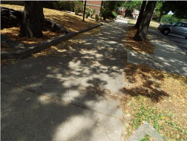
457. Building 12 - sidewalk trip hazards (Critical Repair)
