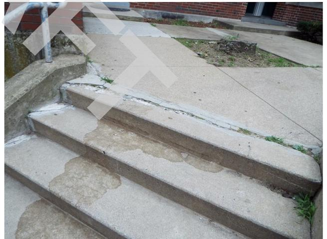
460. Building 12 - concrete stair trip hazard (Critical Repair)
