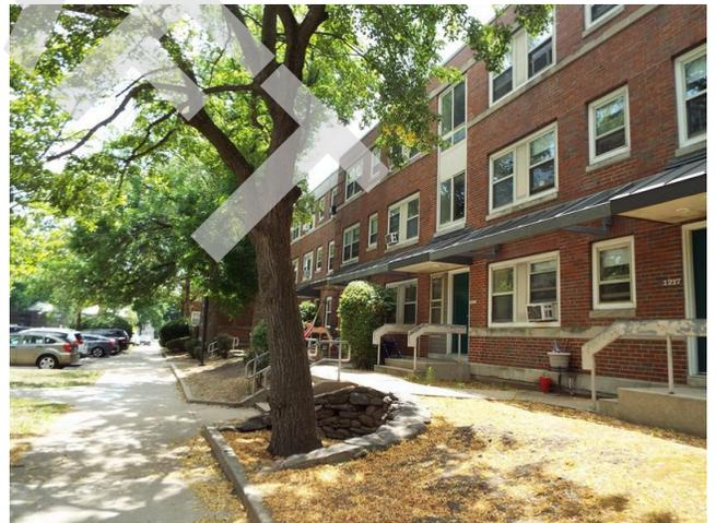
456. Building 12 - stone retaining wall and peeling paint on hand railings (Non-Critical Repair)
