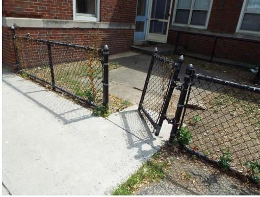
Building 10 - chain link fence damage
