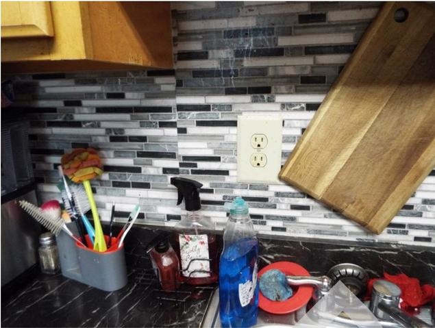
277. Building 12 - unit 1224 - 5-bed/2bath - TH - kitchen missing GFCI (Critical Repair)
