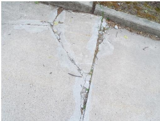
Building 8 - sidewalk trip hazard (Critical Repair)
