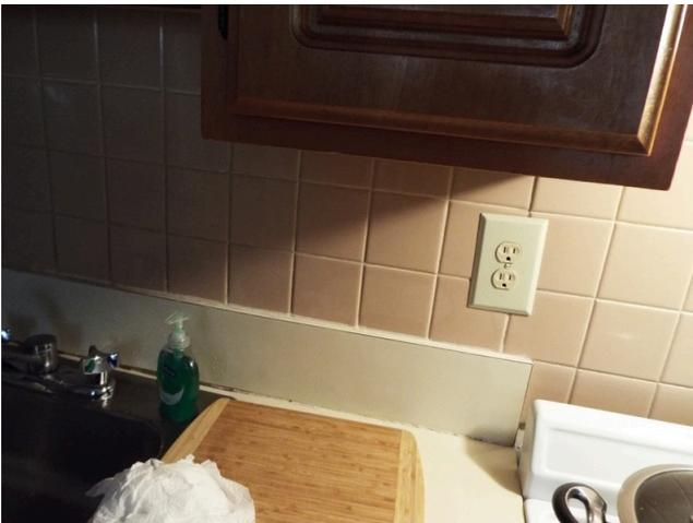
271. Building 12 - unit 1220 - 4-bed/2-bath - TH - kitchen missing GFCI (Critical Repair)
