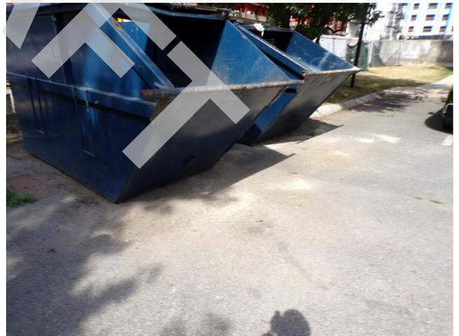
32. Building 4 - dumpsters missing concrete pad
