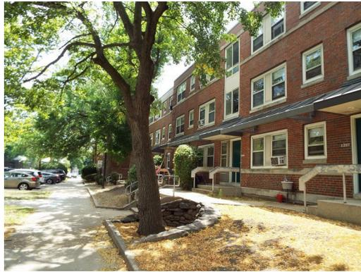
Building 12 - stone retaining wall and peeling paint on hand railings (Non-Critical Repair)
