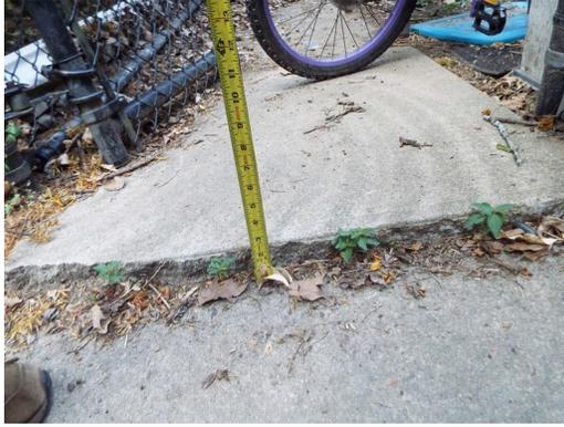
Building 12 - sidewalk trip hazard (Critical Repair)
