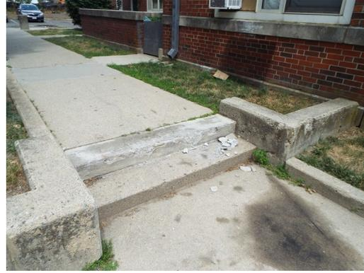
Building 10 and 11 - concrete step trip hazard
