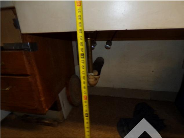
9. Building 4 - unit 414 - 3-bed/2-bath - TH - UFAS - kitchen sink pipes missing scald and abrasion protection (Critical Repair)
