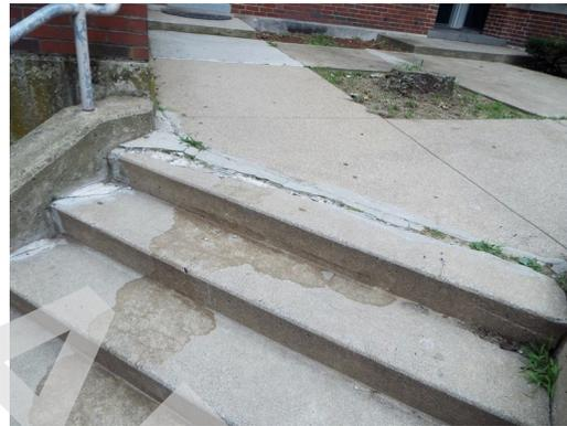
Building 12 - concrete stair trip hazard (Critical Repair)
