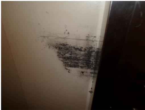
Building 7 - elevator cab door rubbing (Non-Critical Repair)
