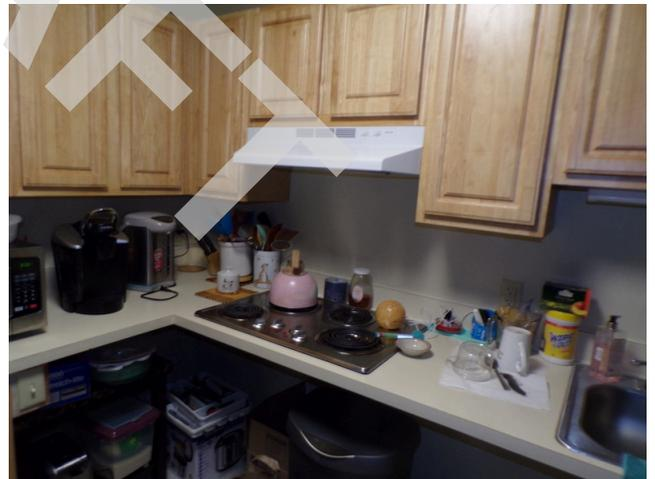
152. Building 4 - unit 417 - 3-bed/1.5-bath - UFAS - kitchen range hood missing front end controls (Critical Repair)
