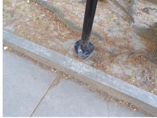
Building 4 - damaged pole light (Non-Critical Repair)
