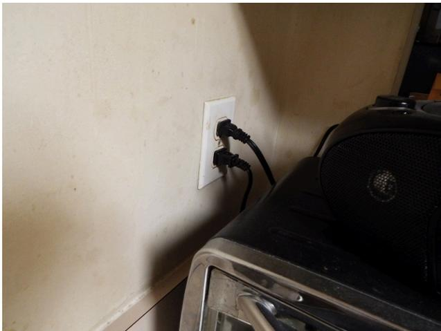
259. Building 11 - unit 1104 - 4-bed/2-bath - TH - unit 1104 - kitchen missing GFCI (Critical Repair)
