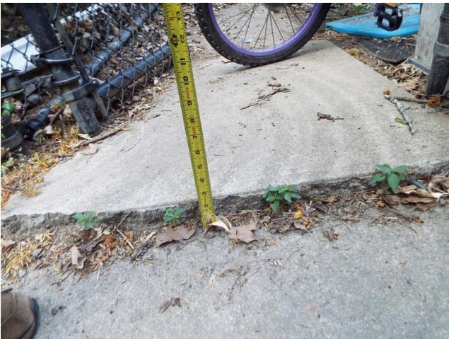
447. Building 12 - sidewalk trip hazard (Critical Repair)
