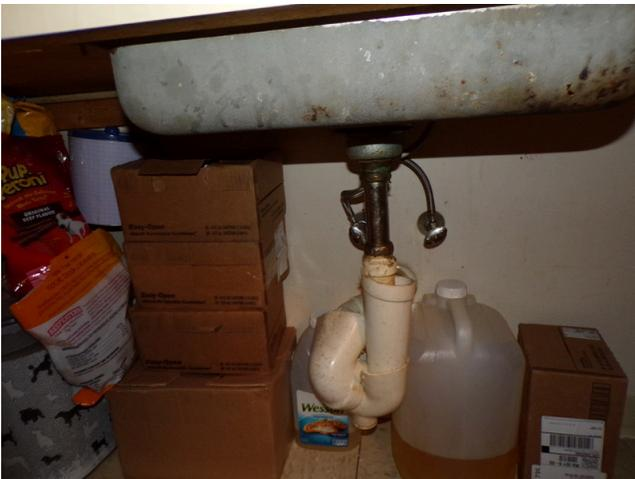
107. Building 4 - unit 432 - 4-bed/1.5-bath - UFAS - kitchen sink missing partial scald and abrasion protection (Critical Repair)
