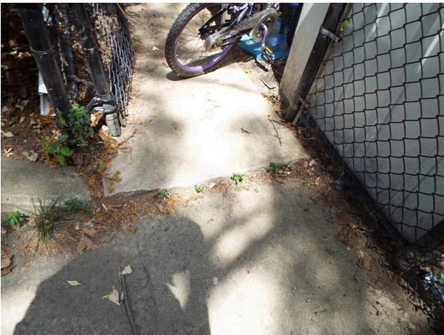
451. Building 12 - sidewalk trip hazard (Critical Repair)
