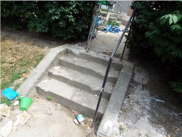
421. Building 10 - concrete stair damage (Critical Repair)
