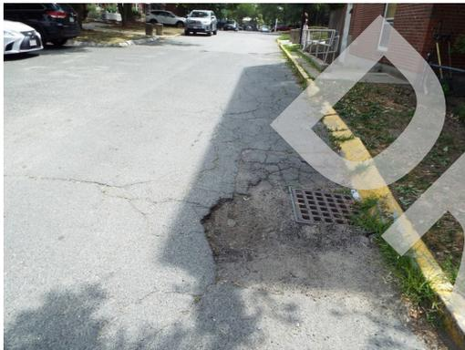
Building 8 - asphalt condition (Non-Critical Repair)
