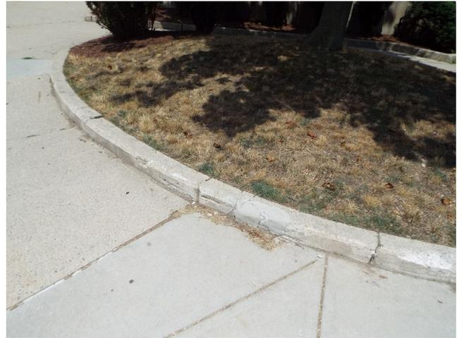
478. Building 13 - curb damage (Non-Critical Repair)
