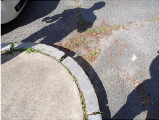
Building 4 - curb damage trip hazard (Critical Repair))
