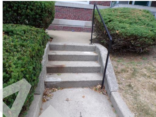
Building 7 - stairs missing railing (Critical Repair)
