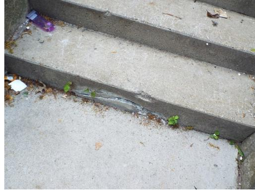
Building 13 - concrete stairs damaged (Critical Repair)
