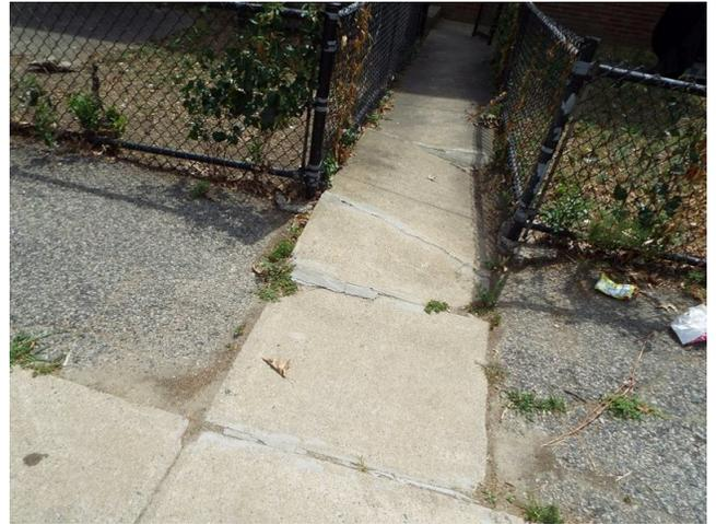
422. Building 10 - sidewalk trip hazard (Critical Repair)
