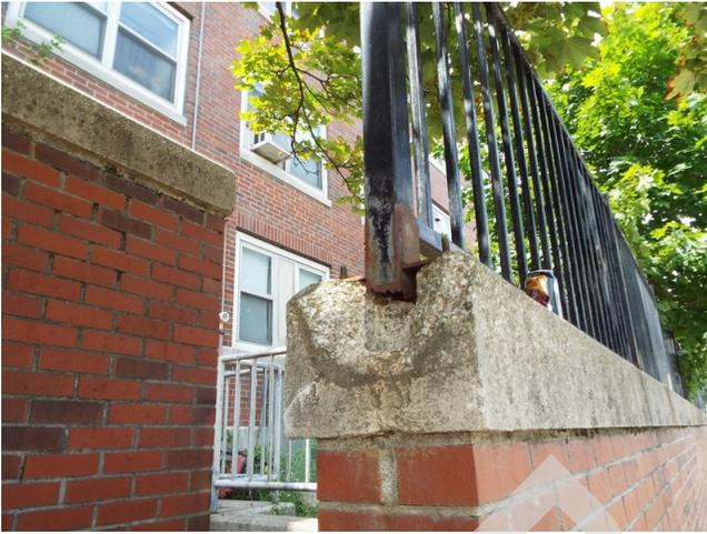
441. Building 11 - retaining wall damage by fence
