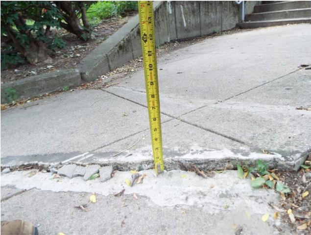
469. Building 13 - sidewalk trip hazard (Critical Repair)
