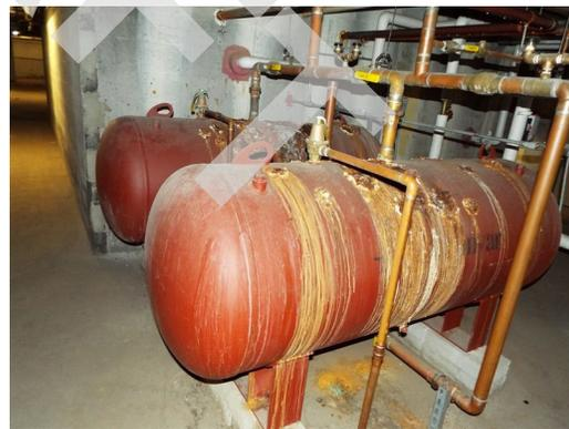
Building 11 - hot water storage tank corrosion
