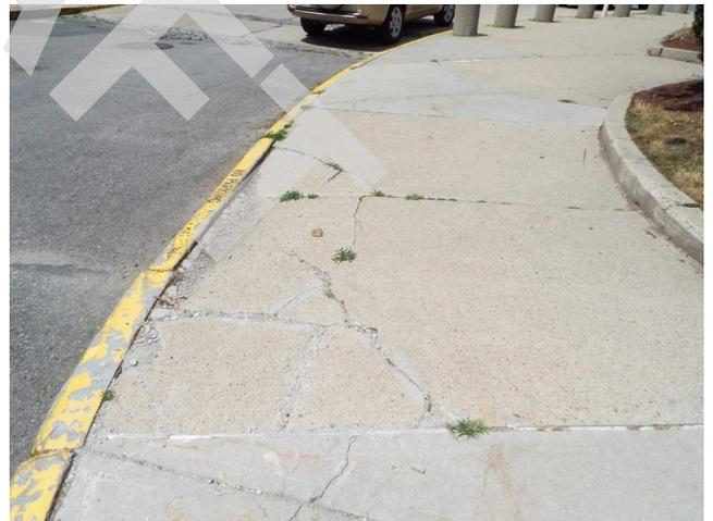
464. Building 13 - sidewalk trip hazard (Critical Repair)
