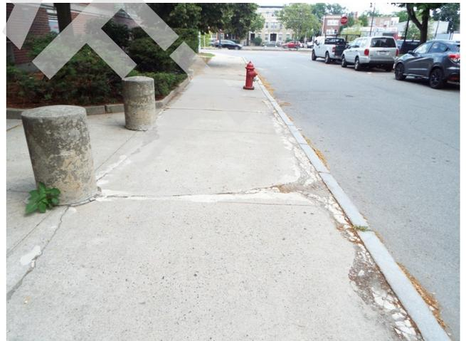
420. Building 10 - sidewalk trip hazard (Critical Repair)
