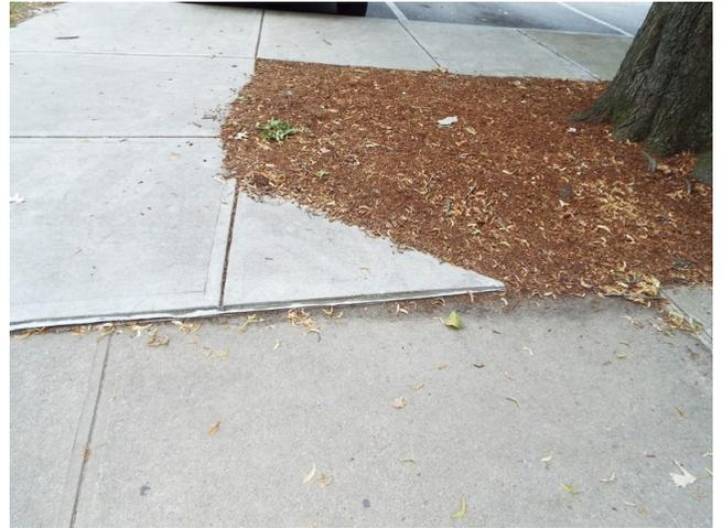
446. Building 12 - sidewalk trip hazard (Critical Repair)
