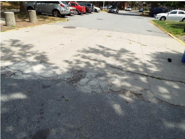
491. Building 13 - damaged concrete sidewalk and paving trip hazard (Critical Repair)
