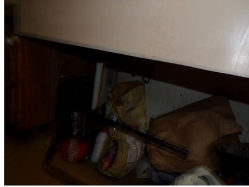
Building 5 - unit 515 - 3-bed/1.5-bath - TH - UFAS - kitchen sink missing scald and abrasion protection (Critical Repair)
