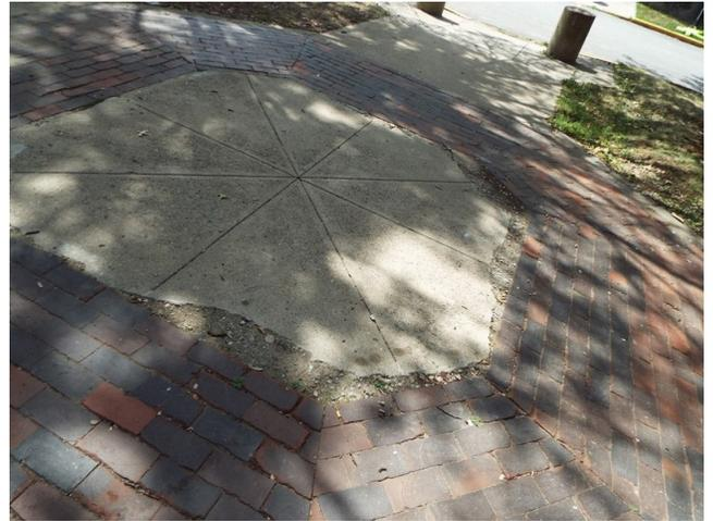
418. Building 9 - sidewalk trip hazard (Critical Repair)
