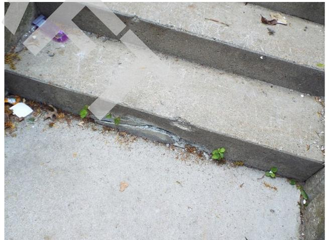
484. Building 13 - concrete stairs damaged (Critical Repair)
