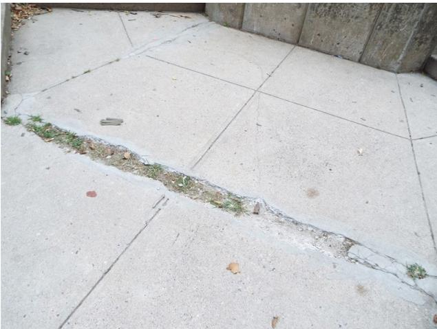
459. Building 12 - sidewalk trip hazard (Critical Repair)
