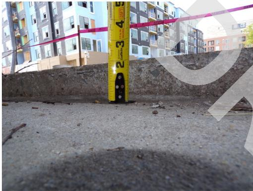
Building 5 - sidewalk trip hazard (Critical Repair)
