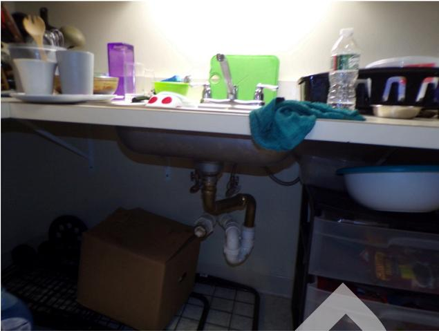
145. Building 4 - unit 437 - 4-bed/1.5-bath - UFAS - kitchen sink missing scald and abrasion protection (Critical Repair)
