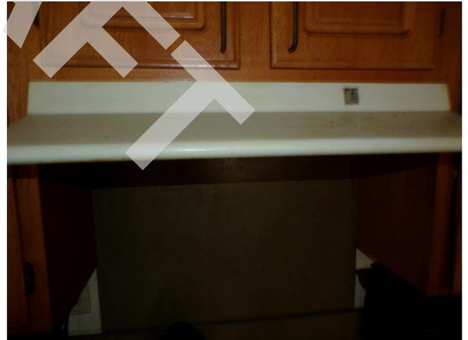
136. Building 4 - unit 427 - 3-bed/1.5-bath - UFAS - kitchen range hood missing front end controls (Critical Repair)
