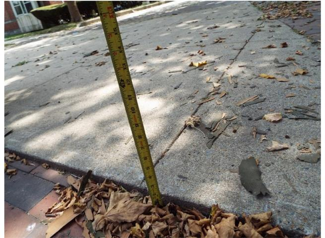
470. Building 13 - sidewalk trip hazard (Critical Repair)
