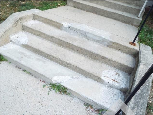
465. Building 13 - concrete stair trip hazard and missing railing (Critical Repair)
