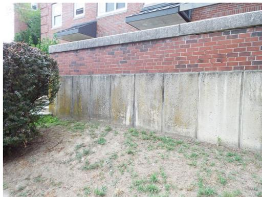
Building 8 - power wash foundation (Non-Critical Repair)
