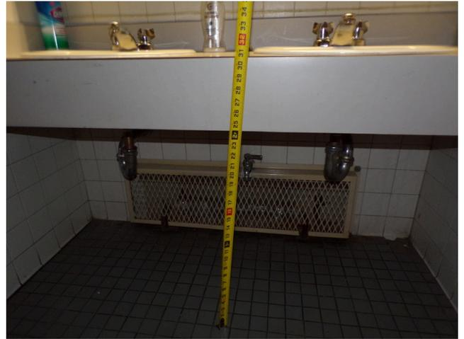
210. Community building - men's restroom missing scald and abrasion protection and levered sink hardware (Critical Repair)
