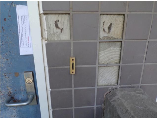
51. Building 4 - unit 418 - 3-bed/1.5-bath - TH - tile damage outside main ingress/egress (Non-Critical Repair)
