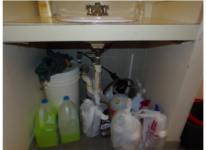
130. Building 4 - unit 415 - 3-bed/2-bath - TH - UFAS - bathroom sink missing scald and abrasion protection (Critical Repair)
