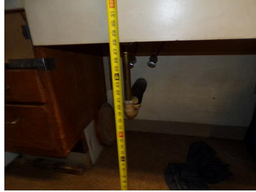
Building 4 - unit 414 - 3-bed/2-bath - TH - UFAS - kitchen sink pipes missing scald and abrasion protection (Critical Repair)
