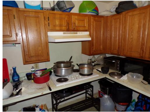
Building 4 - unit 412 - 3-bed/1.5-bath - UFAS - kitchen range hood missing front end controls (Critical Repair)
