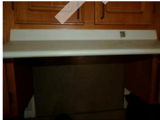
Building 4 - unit 427 - 3-bed/1.5-bath - UFAS - kitchen range hood missing front end controls (Critical Repair)
