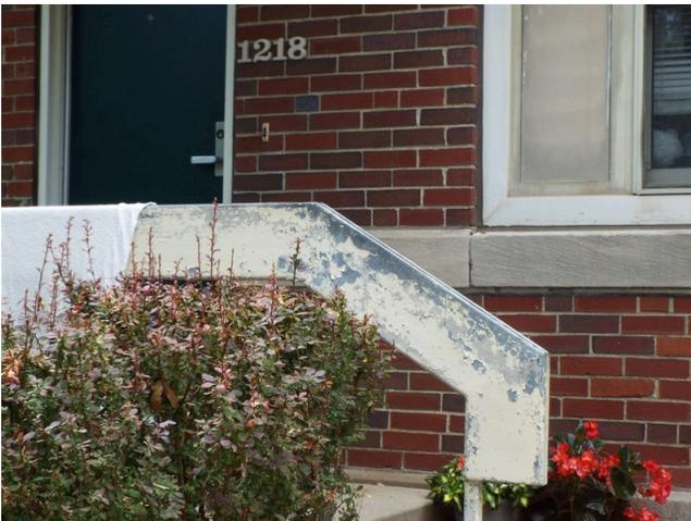
455. Building 12 - peeling paint on hand rail (Non-Critical Repair)
