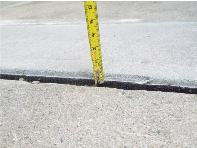
467. Building 13 - sidewalk trip hazard (Critical Repair)
