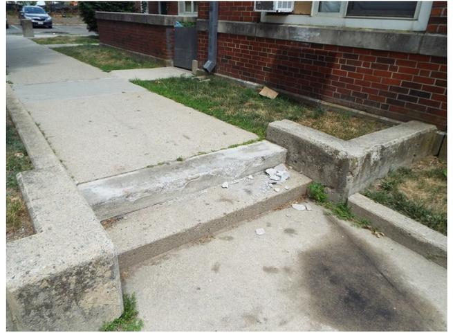
434. Building 10 and 11 - concrete step trip hazard (Critical Repair)
