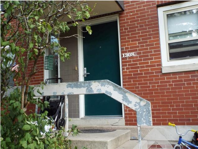
481. Building 13 - handrail paint peeling (Non-Critical Repair)
