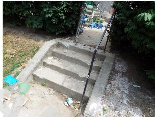
Building 10 - concrete stair damage (Critical Repair)
