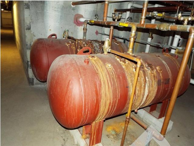
369. Building 11 - hot water storage tank corrosion
