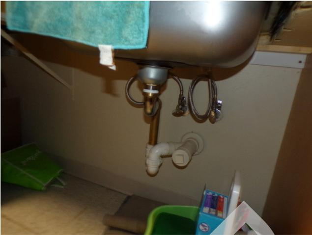
153. Building 4 - unit 417 - 3-bed/1.5-bath - UFAS - kitchen sink missing scald and abrasion protection (Critical Repair)
