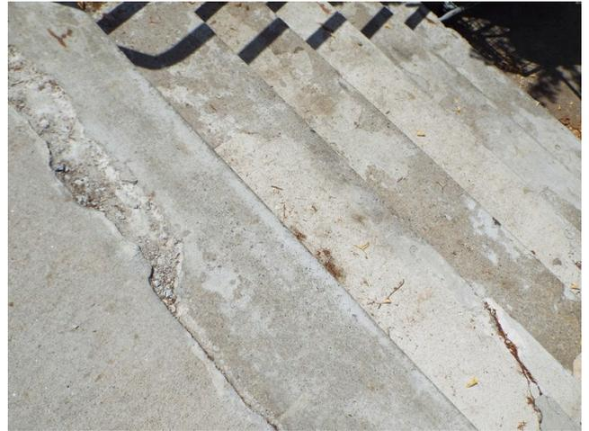
466. Building 13 - concrete stairs trip hazard (Critical Repair)
