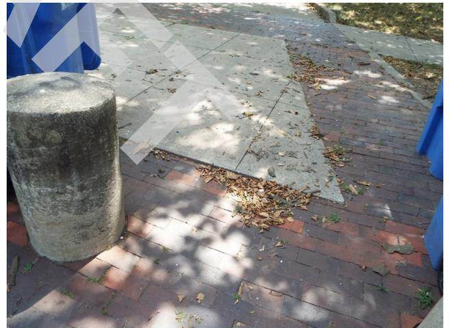
492. Building 13 - sidewalk trip hazard (Critical Repair)
