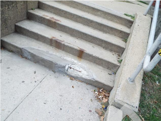
449. Building 12 - concrete steps trip hazard (Critical Repair)
