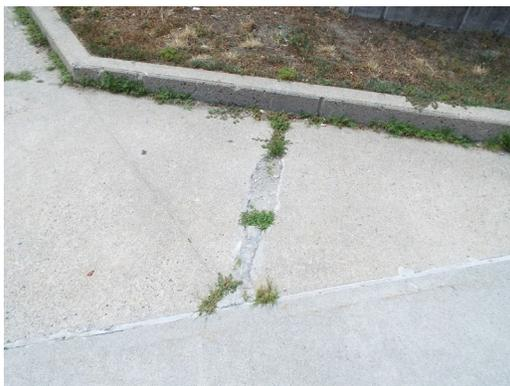
Building 10 - sidewalk trip hazard (Critical Repair)
