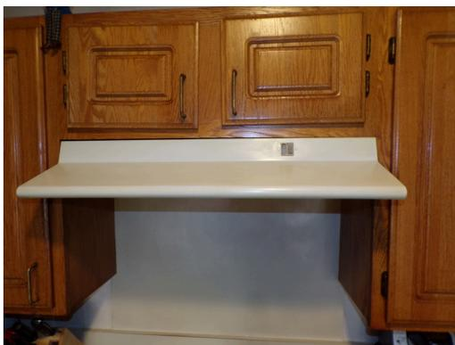
Building 4 - unit 422 - 3-bed/1.5-bath - UFAS - kitchen range hood missing front end controls (Critical Repair)
