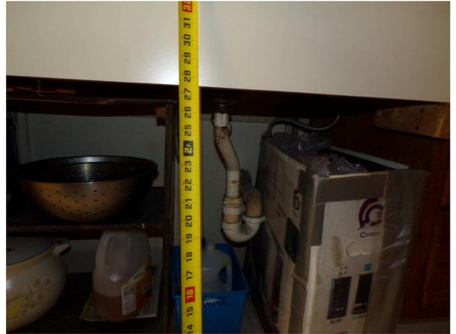
122. Building 4 - unit 415 - 3-bed/2-bath - TH - UFAS - kitchen sink missing scald and abrasion protection (Critical Repair)
