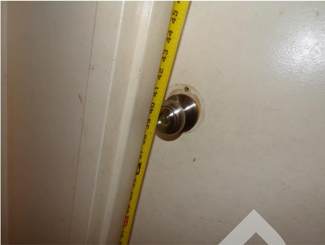
49. Building 4 - unit 412 - 3-bed/1.5-bath - UFAS - non-levered door hardware (Critical Repair)
