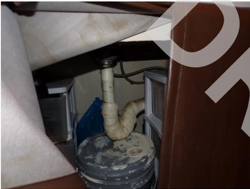
Building 7 - unit 735 - 2-bed/1-bath - UFAS - kitchen sink missing scald and abrasion protection (Critical Repair)
