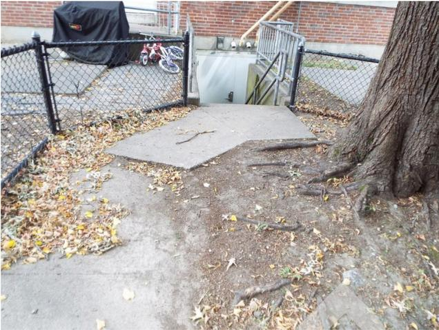
429. Building 10 - sidewalk trip hazard (Critical Repair)
