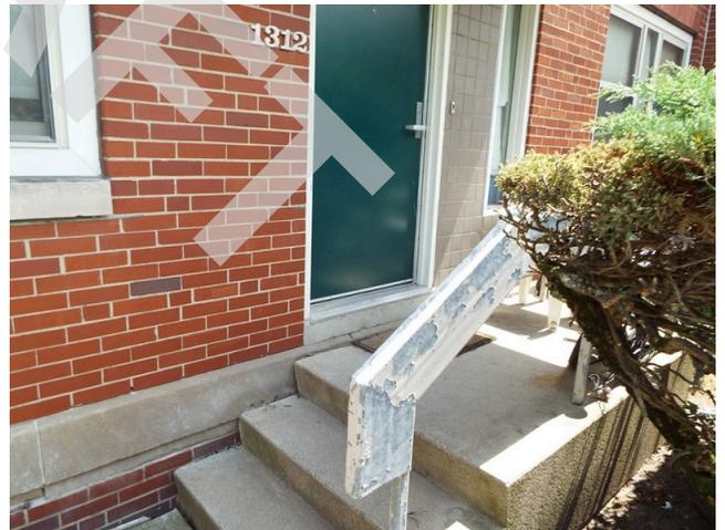
468. Building 13 - hand rail paint peeling (Non-Critical Repair)
