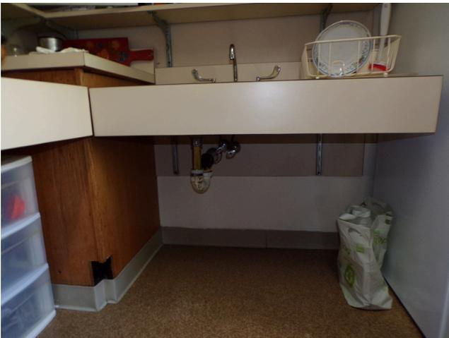
219. Building 7 - unit 731 - 2-bed/1-bath - UFAS - kitchen sink missing scald and abrasion protection (Critical Repair)
