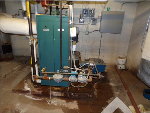
233. Community building - boiler, leak (Critical Repair)
