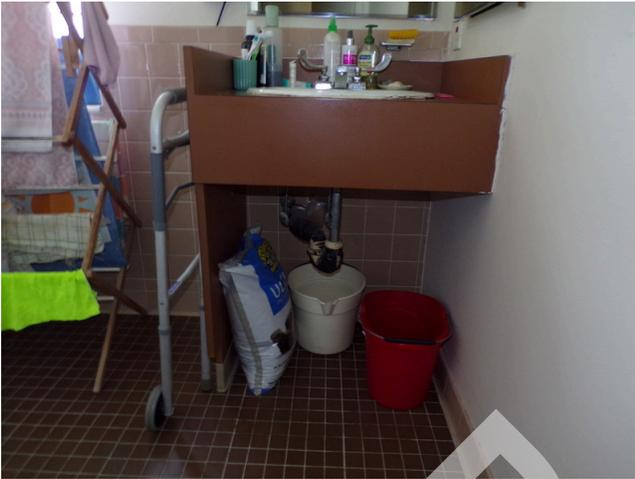
221. Building 7 - unit 731 - 2-bed/1-bath - UFAS - bathroom sink missing scald and abrasion protection (Critical Repair)
