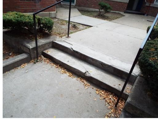
Building 12 - concrete steps trip hazard (Critical Repair)
