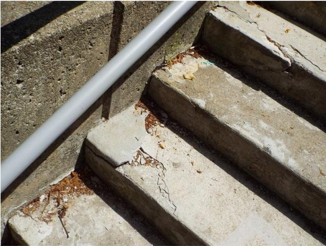
485. Building 13 - concrete stairs trip hazard (Critical Repair)
