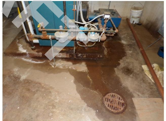
236. Community building - boiler leaking (Critical Repair)
