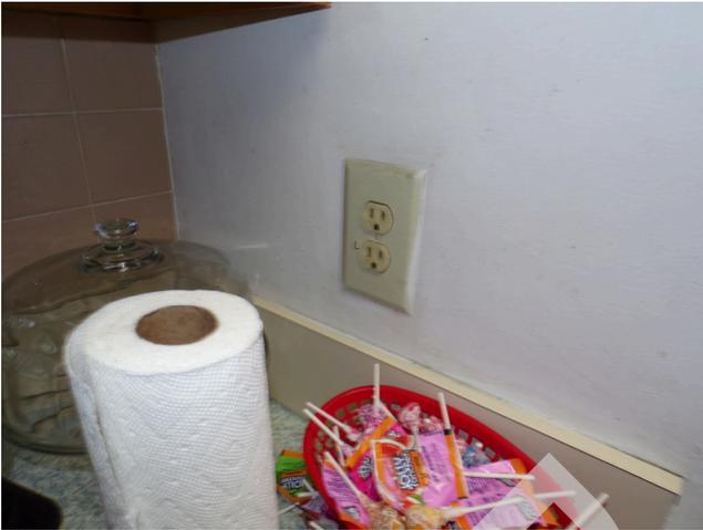
61. Building 4 - unit 418 - 3-bed/1.5-bath - TH - kitchen missing GFCI (Critical Repair)
