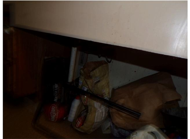
186. Building 5 - unit 515 - 3-bed/1.5-bath - TH - UFAS - kitchen sink missing scald and abrasion protection (Critical Repair)
