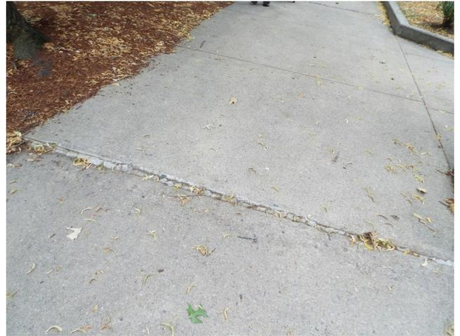
454. Building 12 - sidewalk trip hazard (Critical Repair)
