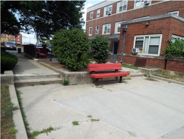
501. Building 10 and 11 - plaza access concrete stairs trip hazard (Critical Repair)
