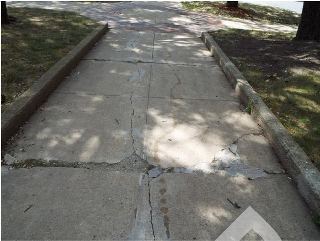
417. Building 9 - sidewalk trip hazard (Critical Repair)
