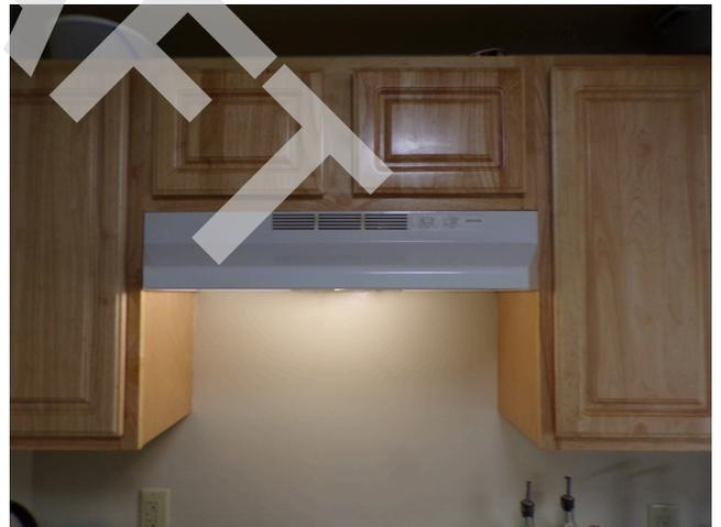
144. Building 4 - unit 437 - 4-bed/1.5-bath - UFAS - kitchen range hood missing front end controls (Critical Repair)
