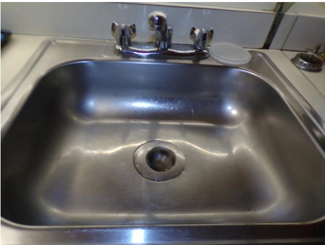
123. Building 4 - unit 415 - 3-bed/2-bath - TH - UFAS - kitchen sink missing levered hardware (Critical Repair)
