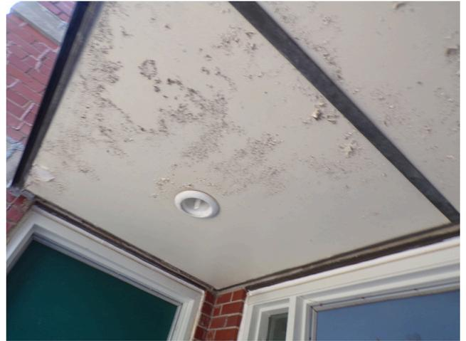
50. Building 4 - unit 418 - 3-bed/1.5-bath - TH overhang paint peeling (Non-Critical Repair)
