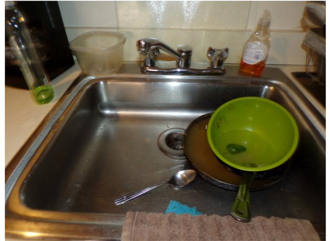
66. Building 4 - unit 422 - 3-bed/1.5-bath - UFAS - kitchen sink missing levered hardware (Critical Repair)
