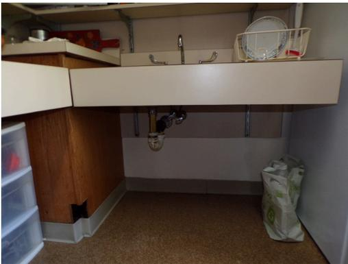
Building 7 - unit 731 - 2-bed/1-bath - UFAS - kitchen sink missing scald and abrasion protection (Critical Repair)
