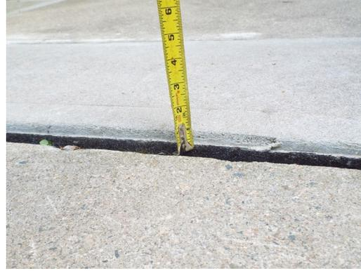
Building 13 - sidewalk trip hazard (Critical Repair)
