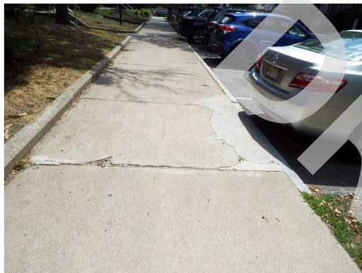
Building 9 - sidewalk trip hazard (Critical Repair)
