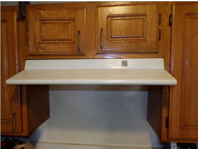
67. Building 4 - unit 422 - 3-bed/1.5-bath - UFAS - kitchen range hood missing front end controls (Critical Repair)
