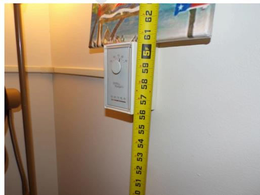
Apartment building 1 - Apartment 111 - 1-bed/1-bath - UFAS unit - heat control thermostat over 48 inches (Critical Repair)
