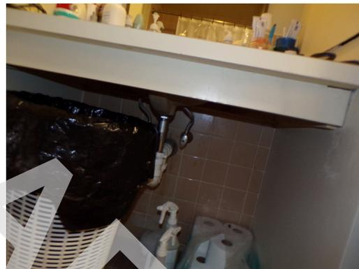
Apartment building 1 - Apartment 114 - 2-bed/1-bath - UFAS unit - bathroom sink missing scald and abrasion protection (Critical Repair)
