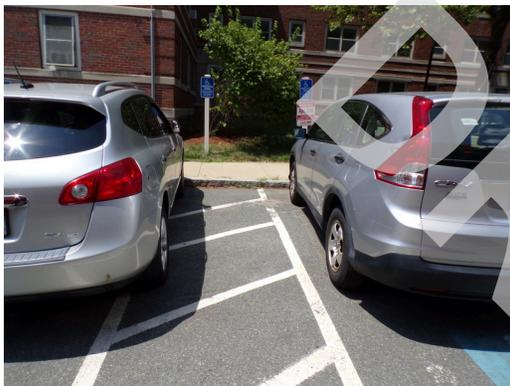
Apartment building 1 handicap parking signage and missing curb cutout (Critical Repair)
