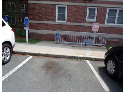
Apartment building 1 handicap parking signage less than 60 inches above ground (Critical Repair)
