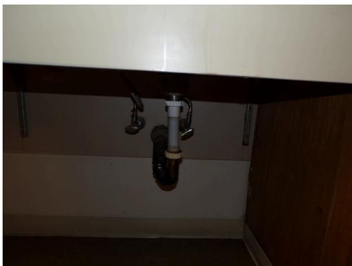
Apartment building 1 - Apartment 111 - 1-bed/1-bath - UFAS unit - kitchen sink missing scald and abrasion protection (Critical Repair)
