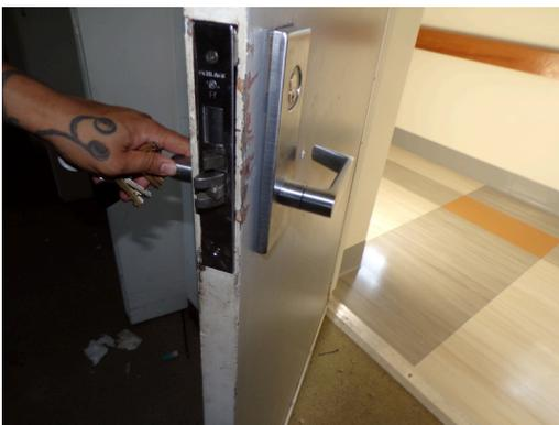
Apartment building 1 - Apartment 145 - 2-bed/1-bath - main ingress/egress door hardware and door condition (Non-Critical Repair)
