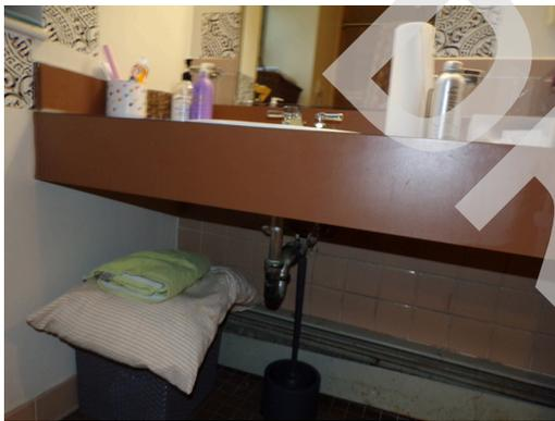
Apartment building 2 - Apartment 212 - 1-bed/1-bath - UFAS unit - bathroom sink missing scald and abrasion protection (Critical Repair)
