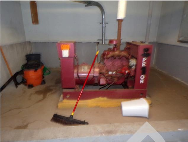
109. Apartment buildings 1 and 2 inoperable fire sprinkler system generator (Critical Repair)
