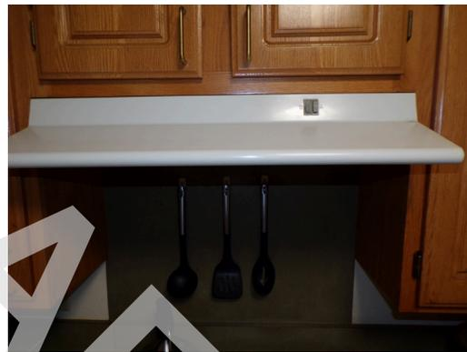
Apartment building 2 - Apartment 214 - 2-bed/1-bath - UFAS unit - Range hood missing front end controls and over 48 inches (Critical Repair)
