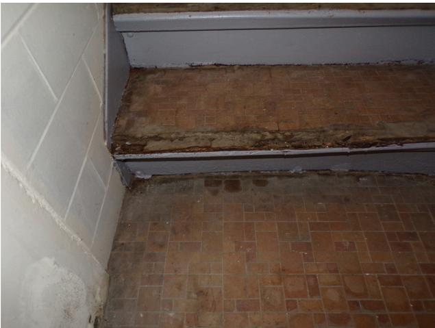
131. Apartment building 1 stairwell B 2nd floor stairs damage trip hazard (Critical Repair)
