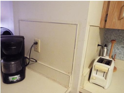
1-bed-1-bath - unit 514 - kitchen lacks GFCI receptacle (Critical Repair)
