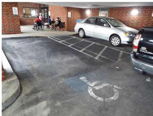
Accessible parking lacks van space and signage (Critical Repair)
