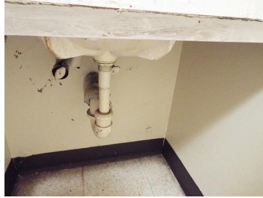
Bathroom sink lacks pipe protection - UFAS -
