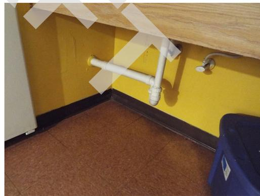
Kitchen sink lacks pipe protection - UFAS - unit 211 (Critical Repair)
