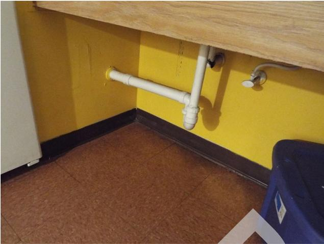
25. Kitchen sink lacks pipe protection - UFAS - unit 211 (Critical Repair)
